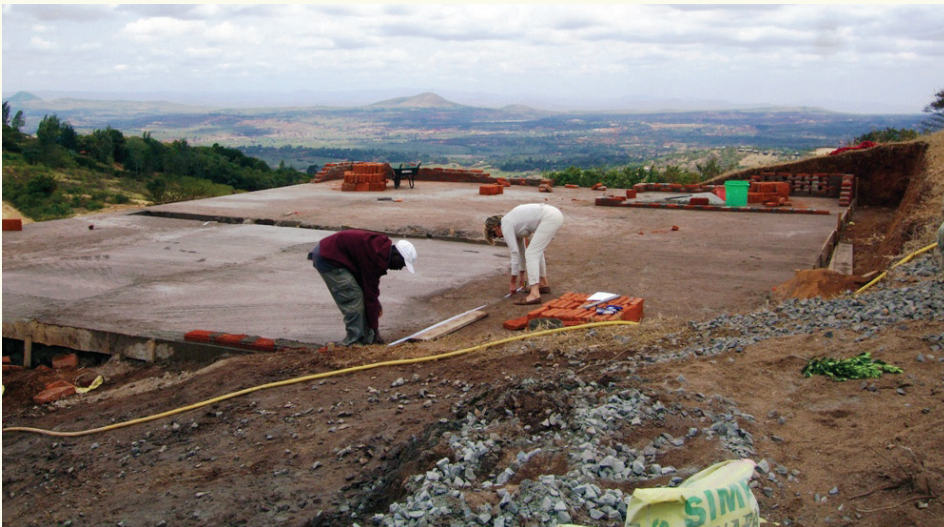
The bakery foundation gets started.
